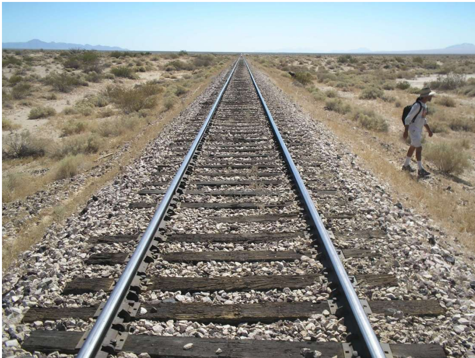
Exhibit G12. View from same location as G11, facing southeast.
