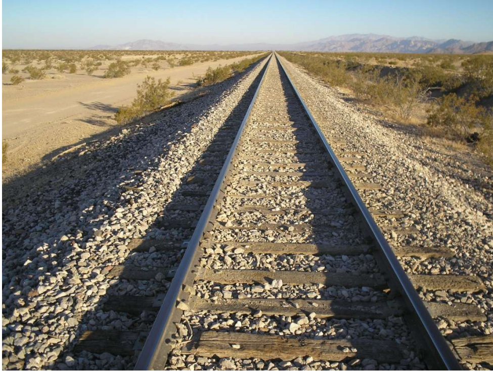
Exhibit G1. View along ARZC ROW, facing north towards Cadiz.
