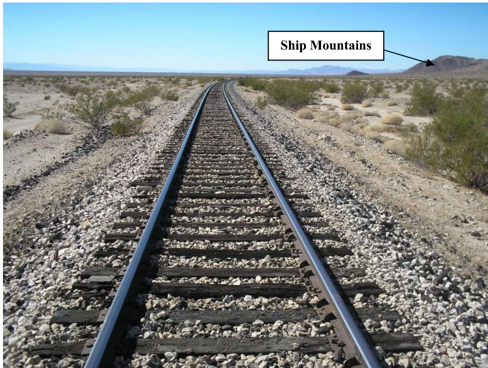
Exhibit G3. View along ARZC ROW, facing north towards Ship Mountains.
