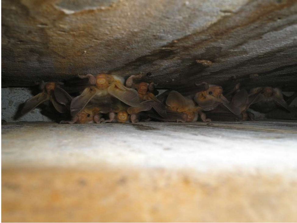
Exhibit I13. Eight pallid bats found in crevice of cement trestle.
